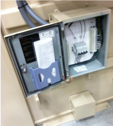
External control box
