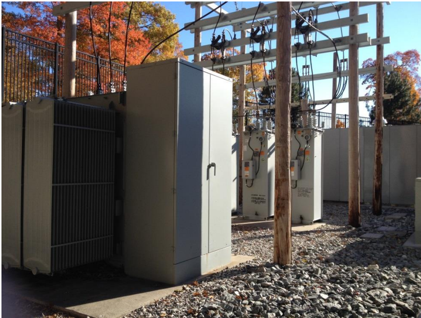
Open type substation and 1-phase regulators
