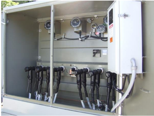
Pad-mounted switchgear
