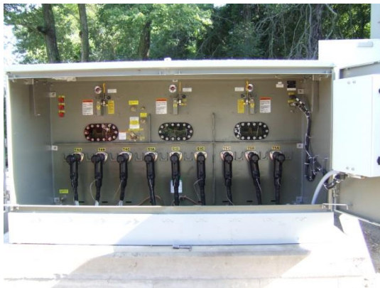
Pad-mounted switchgear
