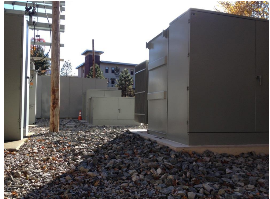
Pad-mounted substation with 3-1 pad-mounted regulator & bypass switch
